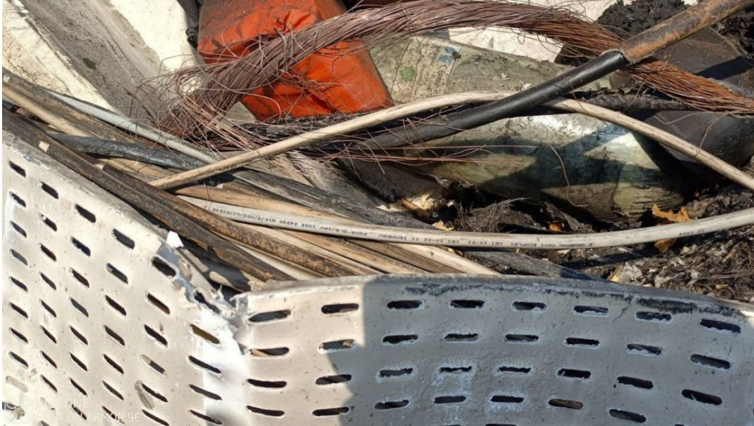
Figure 8. Routing of cable bundles in a metal cable tray (source: AIA)
